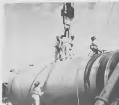
THE TRAVELLING block in position. Mechanical-Yard riggers prepare a huge drum for the lift by the 100-ton gwy derrick. CU E katrol na position, riggers di Mechanical-Yard ta prepara pa hiza un drum grandi door di un gran di 100 ton.
